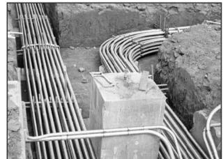
Red brass conduit is most commonly used in swimming pool applications. The rules governing its use are similar to those for rigid steel:
