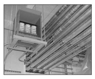
In order for RMC, IMC and EMT to perform effectively as equipment grounding conductors, it is
