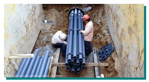
The poem "Invention"<sup>1</sup> illustrates the never-ending quest by the power and communication industries to "get the cord long enough." Conduit-in-casing construction is one method that helps make the cord long enough to get from the communication or power source to the consumer. If you can't go over it, can't go around it and, therefore, need to go under it, conduit-in-casing is often the construction method of choice.
