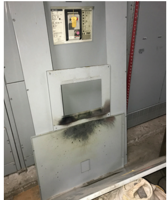
This switchboard could be repaired and/or reconditioned.
