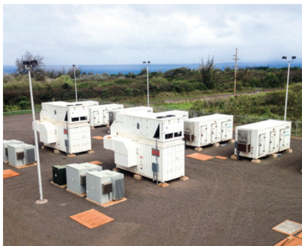
Figure 3. Battery energy storage systems installed by ABB in Hawaii 5
