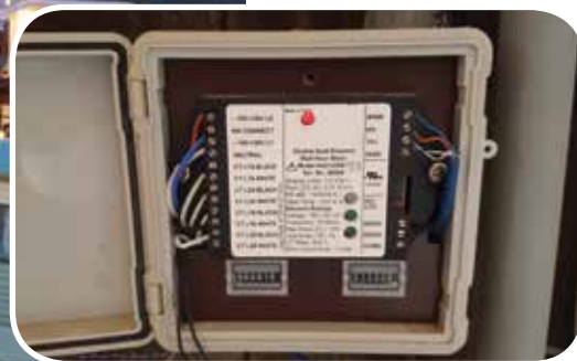
Using submeters to bill end users reduces overall consumption and waste. Submeter photo courtesy of EZ Meter
