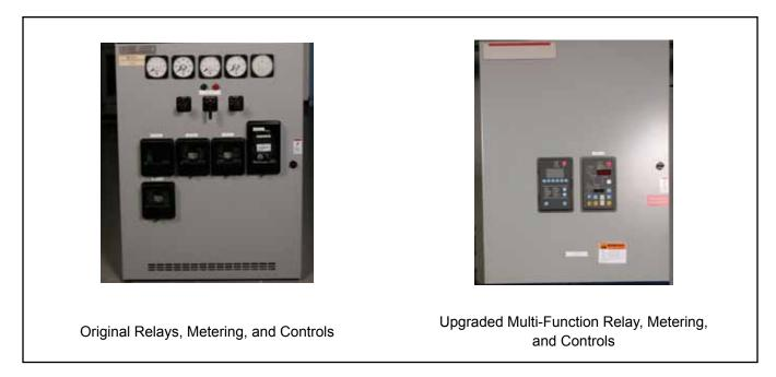
Figure 3. Power Equipment—Protective Relay, Metering, and Controls Upgrade Option
