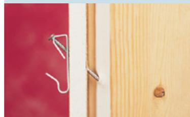
Nonmetallic sheathed cable damaged by gusset plate while being pulled through attic.
