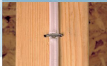
Wires located behind walls can be accidentally punctured by a screw or drill bit damaging the insulation of the wiring.
