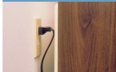
Extension or appliance cords that are damaged or have worn or cracked insulation can contribute to electrical arcing.
