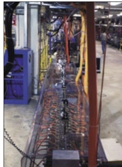
A view down the pipe view (the beam goes down the middle) of the infrared wiggler. Courtesy of Jefferson Labs.
