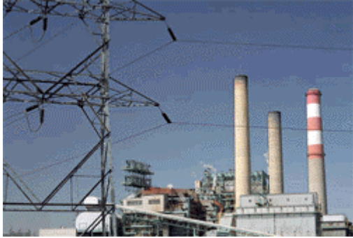
Electrical transmission lines in front of a coal-fired power plant
