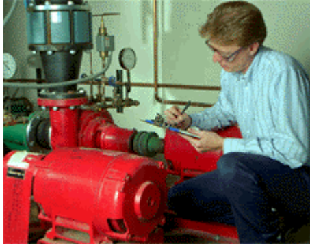
Replacing an inefficient motor
