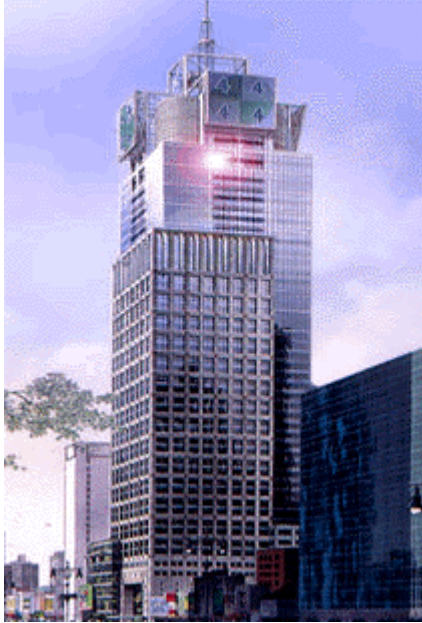
4 Times Square: The first building built in New York in the 1990s, using modern energy efficiency guidelines
